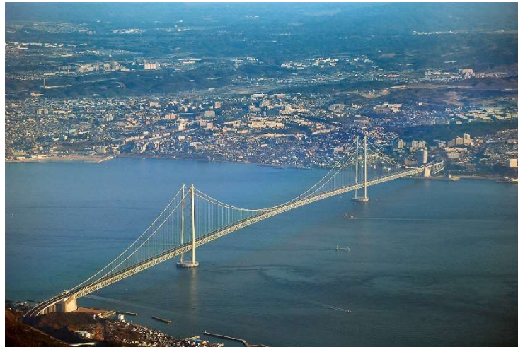
Figure 1: Akashi Kaikyō Bridge – Kobe, Japan
